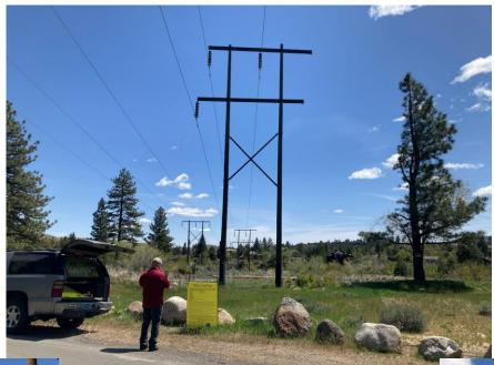
Western Bridge St. Corridor Pole on right side of photo to be removed and replaced with joint circuited poles
